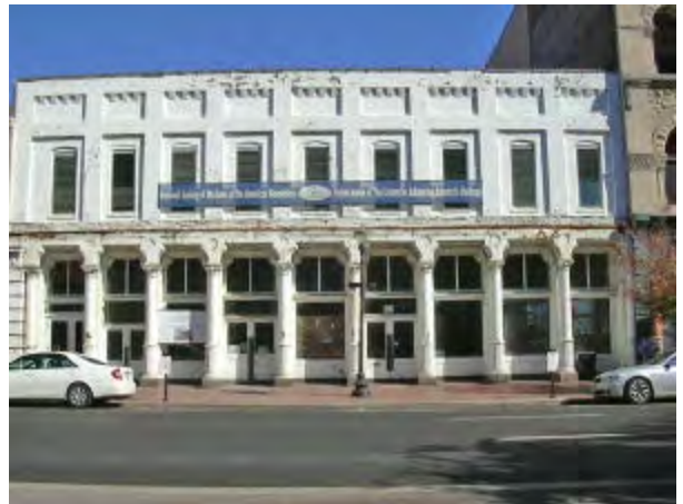
New SAR Headquarters located on East Main in Louisville, KY. This photo is taken looking south at the building.
